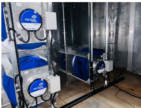
Energy efficient EC Blower at
